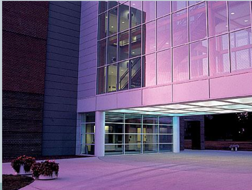
Haenicke Hall, science research laboratory facility Western Michigan University
